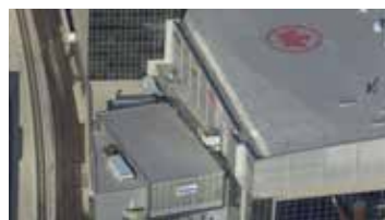
Air Canada Operations Centre, Brampton
